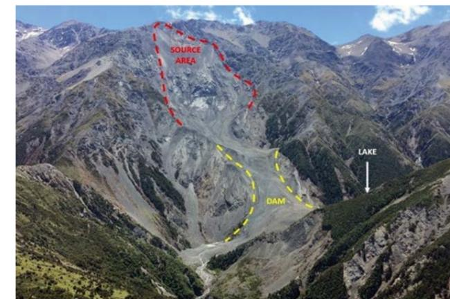
Hapuku landslide dam: about 20 million cubic metres of rock travelled 2.7km to the valley floor. (Photo GNS Science)
